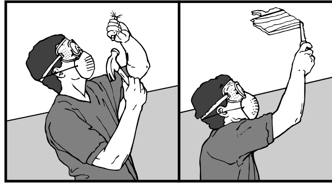
Figure 5. Make a starter hole near the center of the chosen location.
